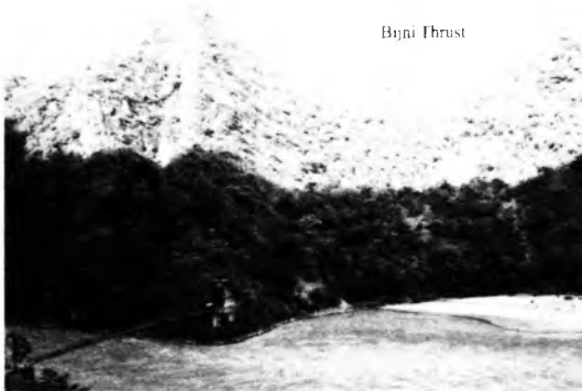
Photo1: Overall View of Thrust Zone as depression near the Power House Ridge
